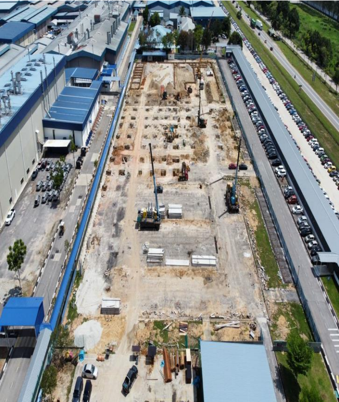
Projek Inokom – Paint Shop (PS3)
