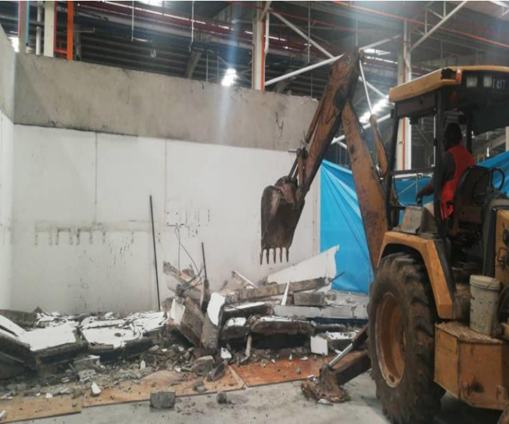
Projek Inokom – BMW Wall Demolish
