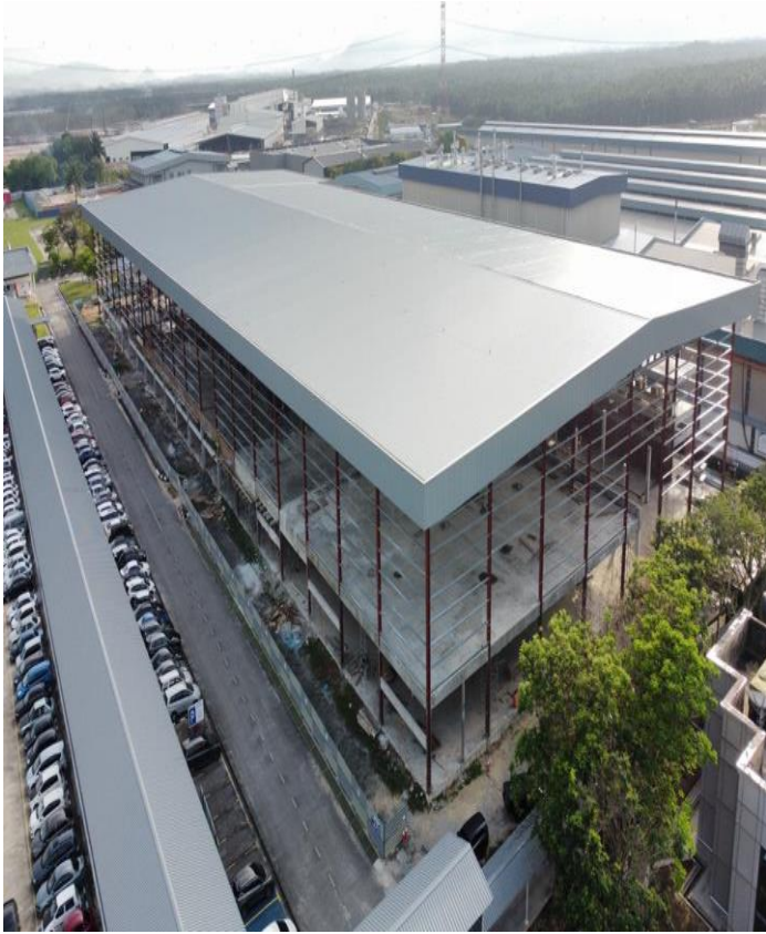
Projek Inokom – Paint Shop (PS3)
